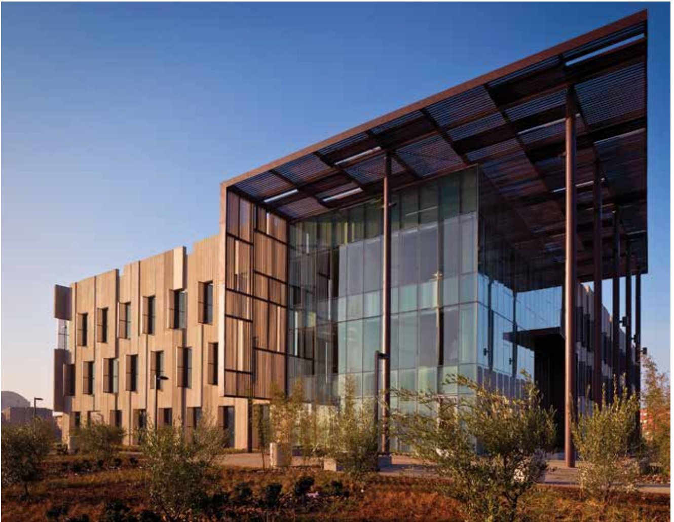
Precast concrete components used on the East Campus Office Building on the campus of the University of California-San Diego helped reduce the budget by serving as both the cladding and the structure. Photo: Ryan Gobuty / Gensler.
